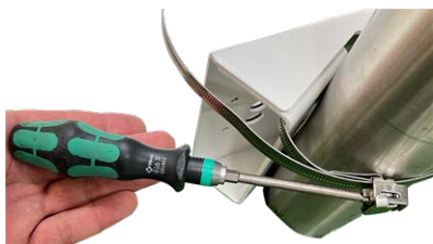
Fig. 14: Tighten the straps
